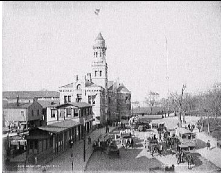
The Barge Office Temporary Immigration Station, circa 1890
